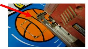
Place Masking tape on the front of the hole.
