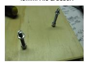
37 - Insert the allthread support legs, with the screw driver slot up, into the pre threaded wooden base.
